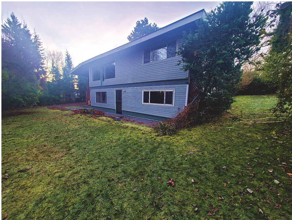
Image 1. Overall view from northwest to southeast.
